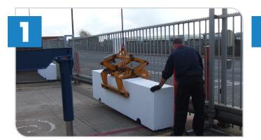
Plan where you want the barriers to be positioned and position close to their final position using a forklift truck.
